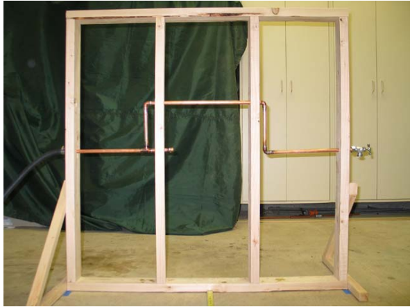
Figure 1 – Test wall before installation of sheet rock
